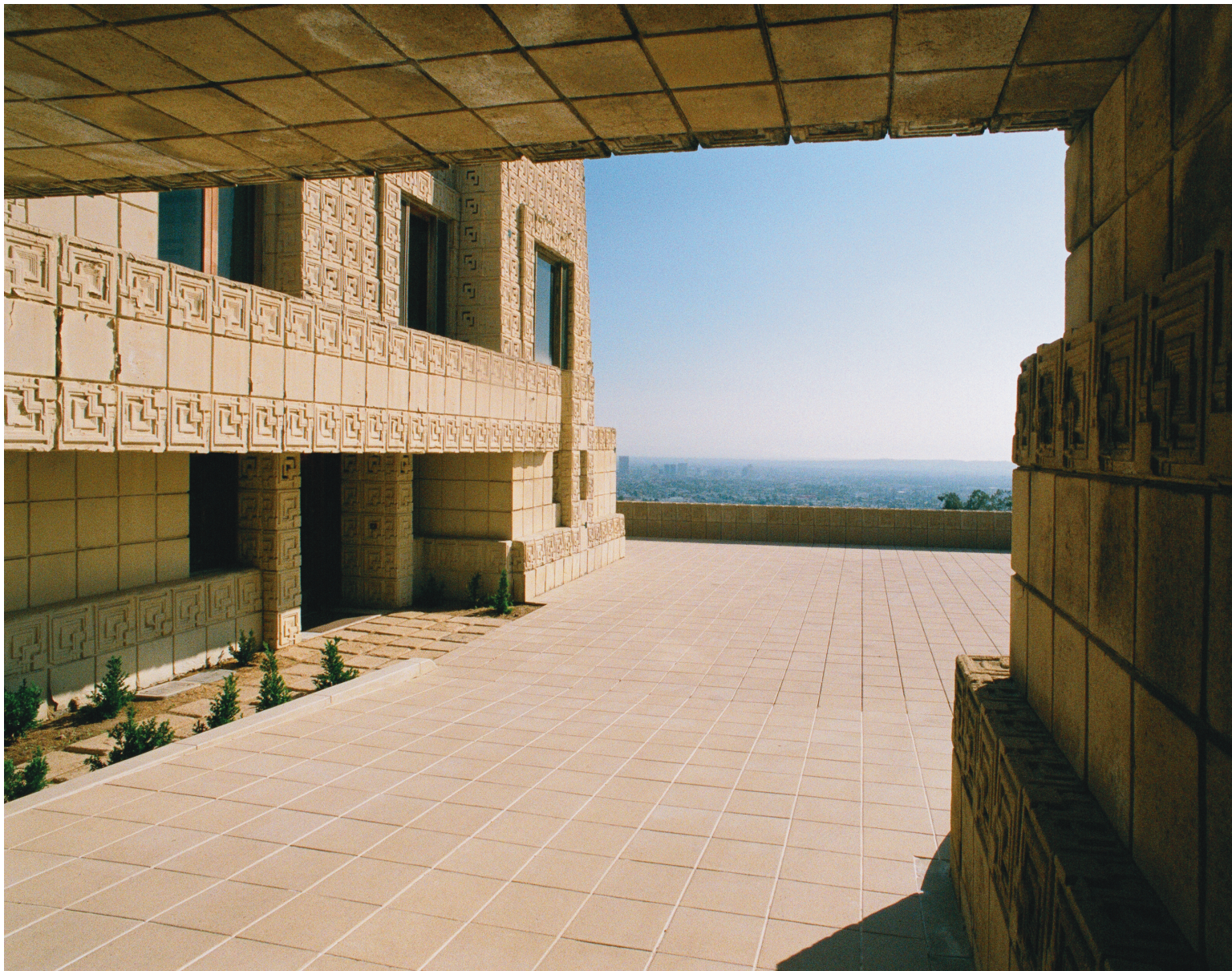
Entrance driveway opens to completely reconstructed motor court — historically correct pavers supported on massive concrete frame replace 80-year old concrete slab formerly resting on earth. Photographic image © Sandra Williams
