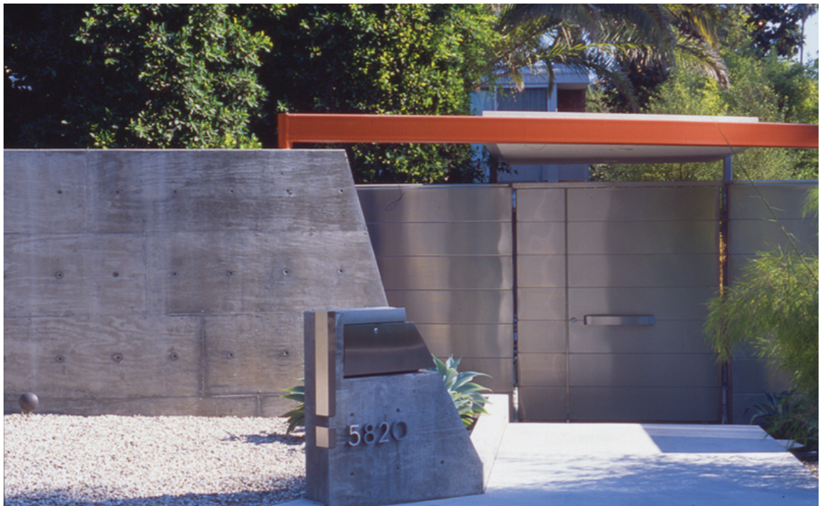
Top — View of restored main building from just inside new front gate; Below — new concrete wall and stainless steel gate. All images © Sandra Williams
