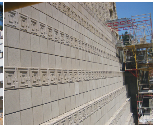
Left — construction of combination precast and poured-in-place concrete foundation and frame; Center — placement of precast concrete wall beams; Right — construction of concrete "textile block" wall to exactly match original wall that had deteriorated beyond repair. Construction images © Wiehle-Carr
